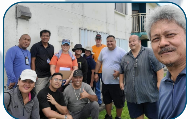
GHC Staff participated in a day long assessment of the condition of GHC rental units in Lada Gardens and Sagan Linahan, Dededo and Guma As-Atdas in Yigo after the passage of Super Typhoon Mawar.
